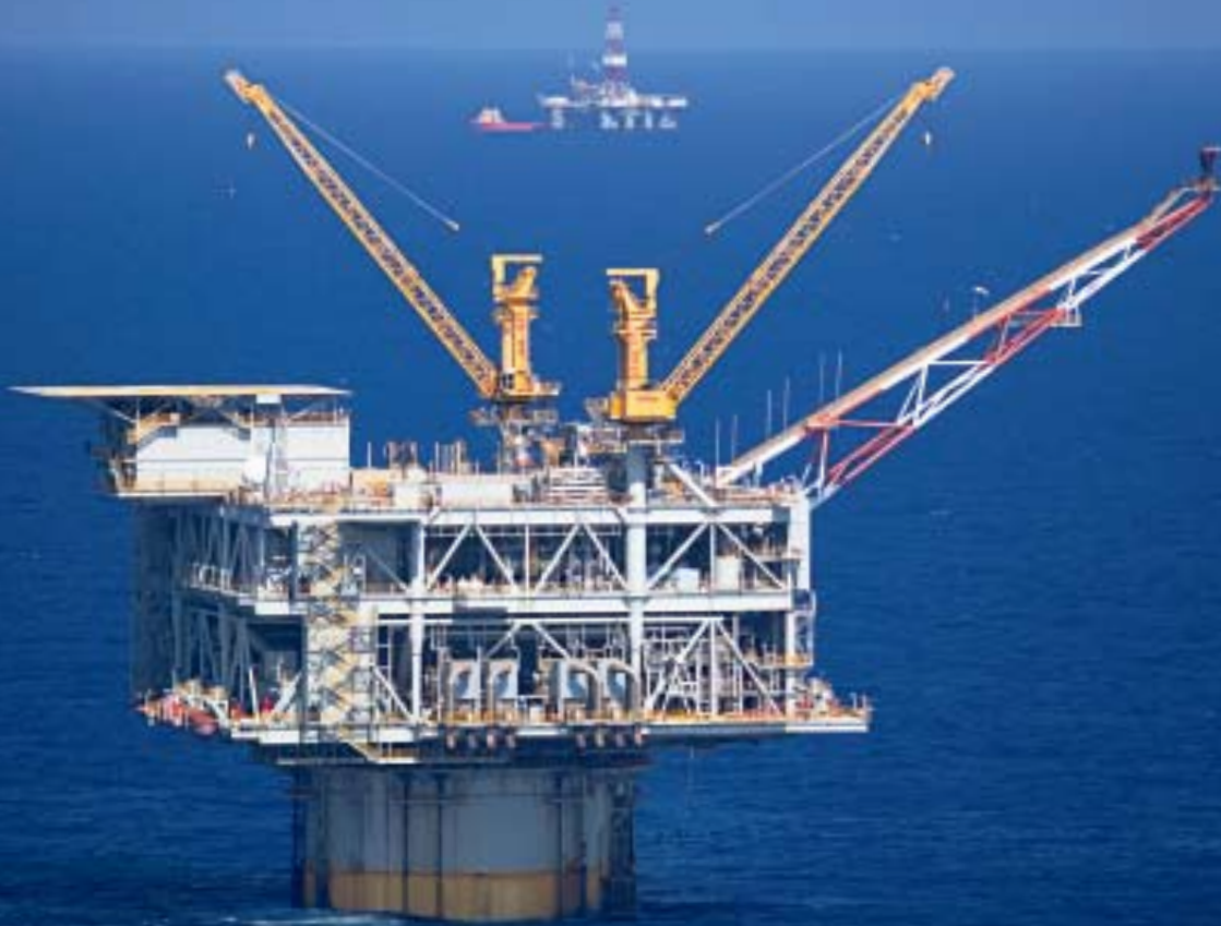
The drillship Ocean Valiant (shown in distance) completed the Rockefeller well in water about a mile deep in three months to a total depth of more than 13,800 feet.
